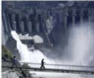
On the edge: Several under-construction developments could risk turning into 'stranded assets' if costs escalated, as
