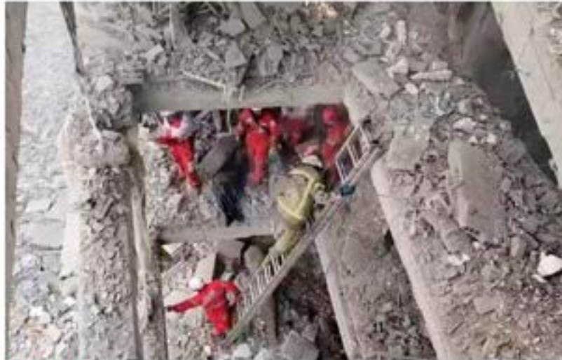
Hit hard: Rescuers work in the rubble of residential buildings after air strikes hit Tehran on Monday. REUTERS
